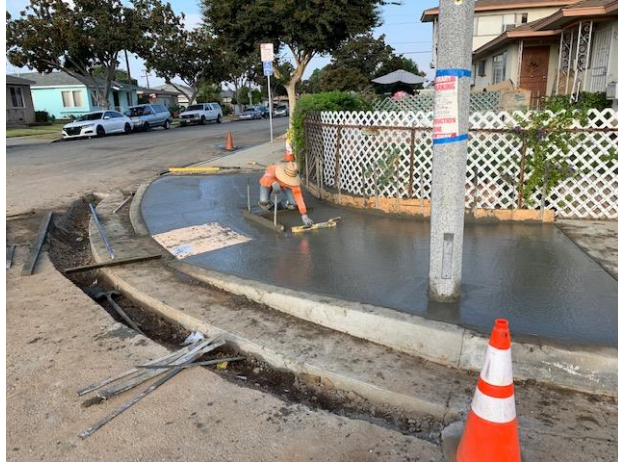
NE corner of Bradley & Beverly Terrace
